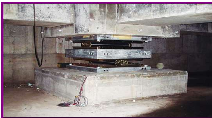
Fig 4: Roller & Ball Bearing Based Isolated Structure
