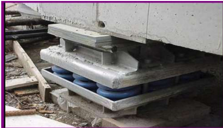
Fig6: Steel Spring Based Isolated Structure
