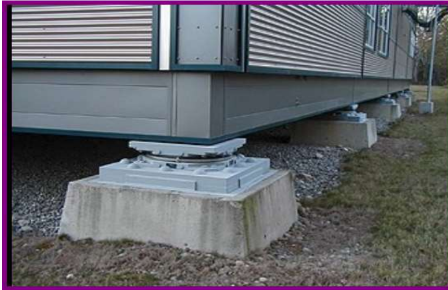
Fig5: Sliding Bearing Based Isolated Structure
